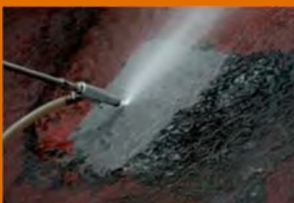
Surface sand blasting
