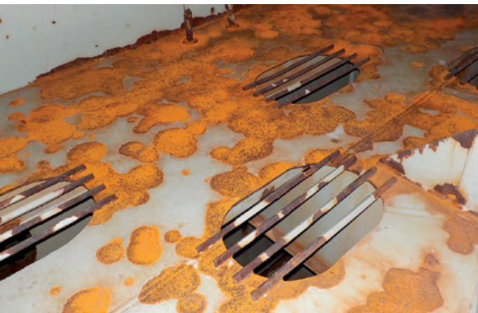
Light flush rust after waterblasting WJ-2 (1800 bar)
