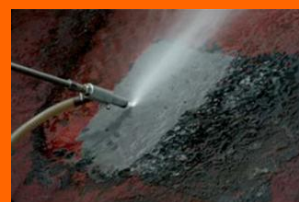
Surface - Sand Blasting
