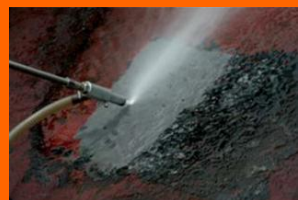
Surface – Sand Blasting
