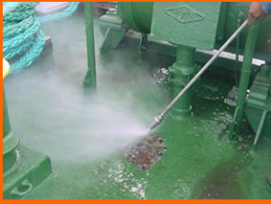
Blasting - Rotating Nozzle
