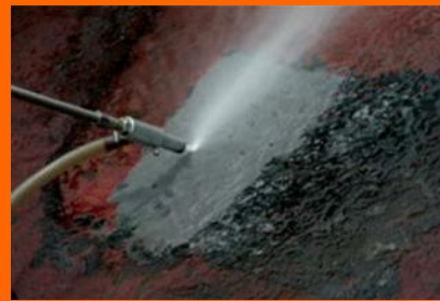
Surface - Sand Blasting
