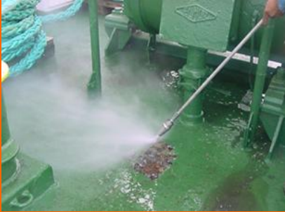
Blasting - Rotating Nozzle
