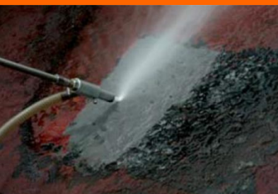
Surface – Sand blasting
