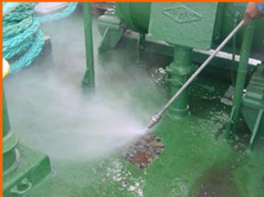
Blasting- Rotating Nozzle
